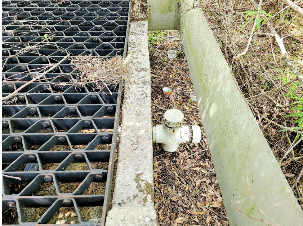
Pond #AA1 Buildup of silt around the existing intake of orifice.
