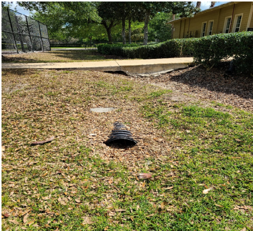
Sidewalk between amenity center and tennis courts – Remove silt and leaves from existing culvert. Place compacted fill 2' out from sidewalk and taper down and sod all disturbed areas.
